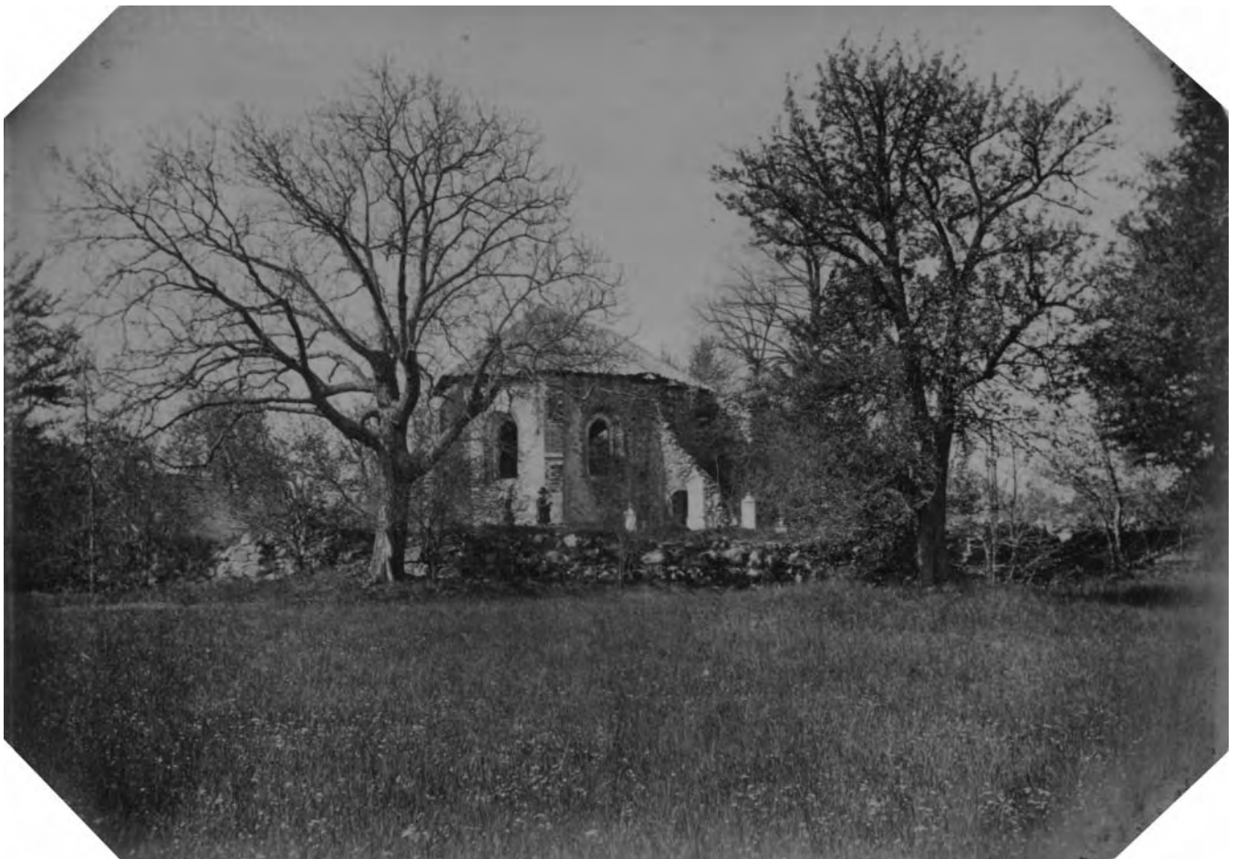
8. Ruins of the church in the Mountain Park, the latter part of the 19th century
