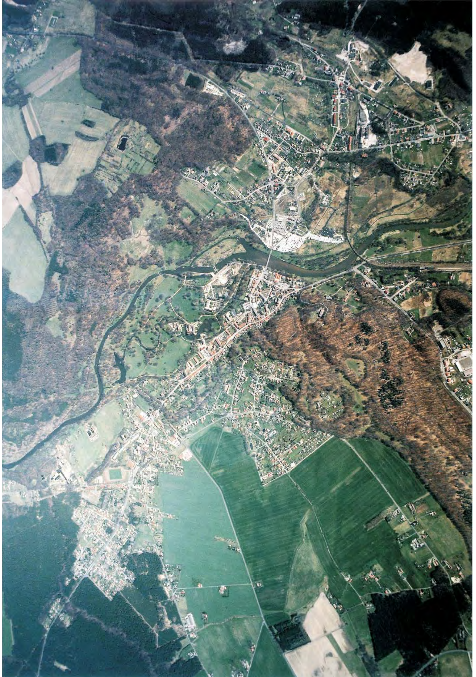
2. Aerial photograph of the park, 2001
